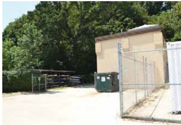
Existing Sanitary Pumping Station
