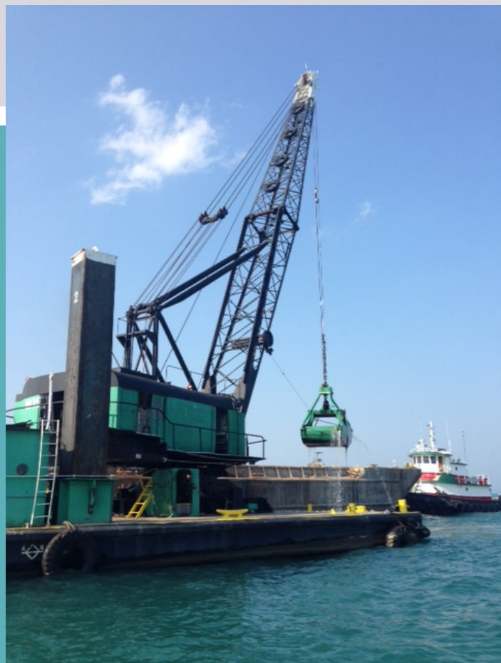
Above: Dredging in the Waukegan Harbor Approach Channel (IDNR, 2015)
